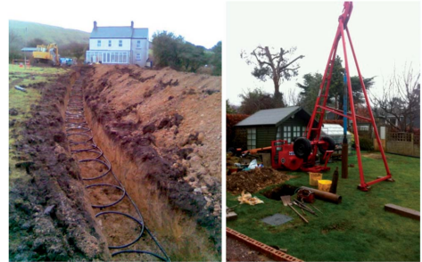
Fig. 6 The installation of ground loops for GSHP systems using slinky horizontal pipes (left) and a vertical borehole (right). Source: Staffell et al, 2012
